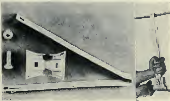
Fig. 4.—Special design trolley wire hanger.
